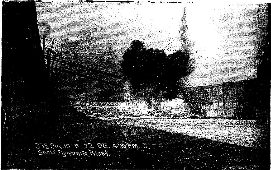
Photograph taken in 1895 during the excavation of the Chicago Sanitary and Ship Canal. Notice the steep vertical walls on the sides of the channel.
